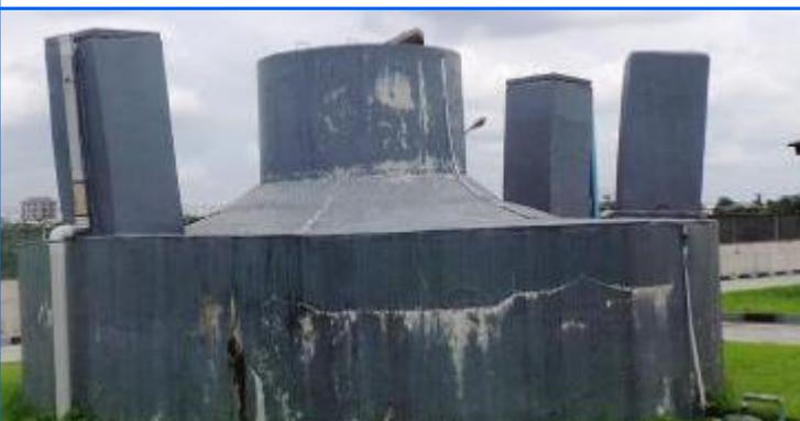
The dome shape structure here shows an anaerobic digester where the anaerobic treatment process is carried out. The anaerobic digester process of Port Harcourt Water corporation Waste Water Treatment Plant at Eagle Island has been scaled up for the production of Methane Gas for cooking and other allied uses. PHWC is strategizing on the process of making the process viable and sustainable for the generation of much needed revenue to fund its operations and support the Government of rivers state.
