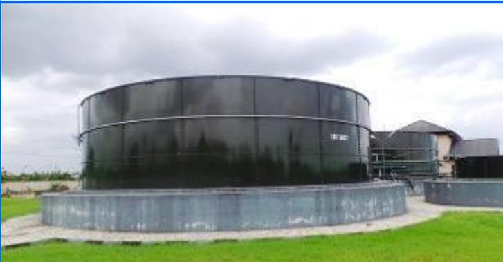
Wastewater treatment can be achieved by biological process either through an aerobic process or anaerobic process. In the WWTP at Eagle Island, we have both systems available. The tank in the adjoining picture shows a Sequence Batch Reactor (SBR) where aerobic process is carried out with some flocculants are added to aid solid liquid separation.
